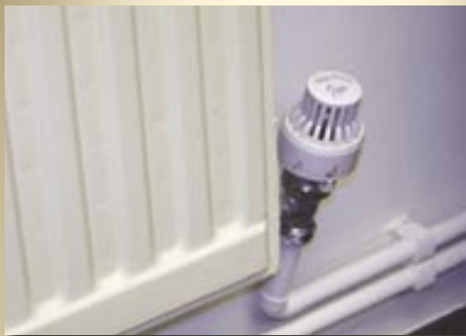
Radiator edges, valves and exposed pipework are a potential hazard
