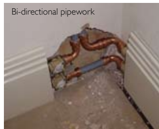
Using threshold kit on solid floor
